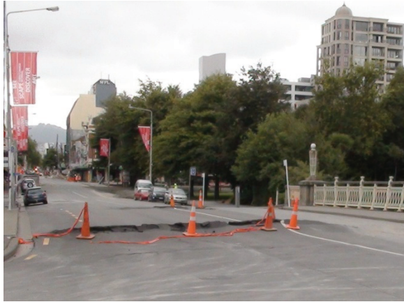
Figure 22 – Colombo Street bridge (a) Slumping of riverbank close to bridge; (b) Buckling of fascia arches; (c) Slumping of abutments at end of bridge; (d) Undamaged straight riveted girders. (Leon)
