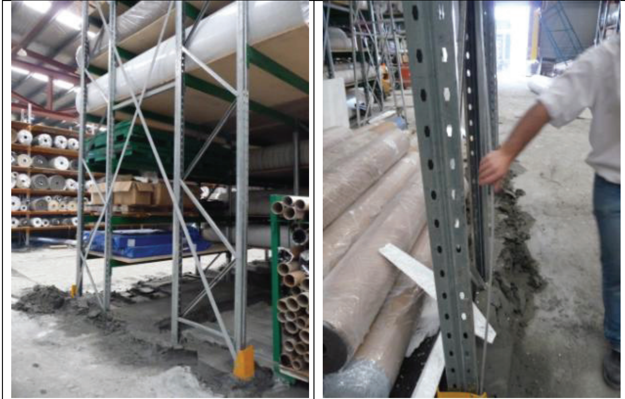
Figure 15: Industrial storage racks that survived, with evidence of soil liquefaction [Photos by M. Bruneau]; (a) Global view; (b) Close –up of buckled brace.
