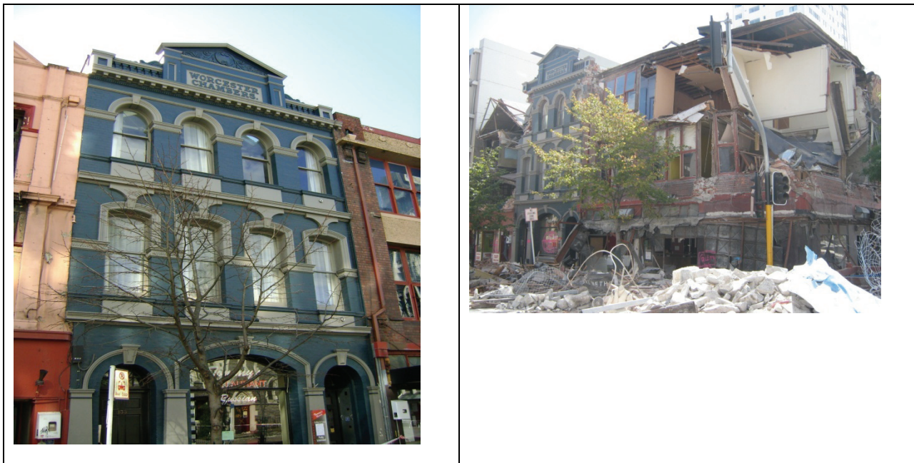
Figure 12: Strengthened URM buildings: (a) is following the September 2010 event and (b) following the February 2011 event, taken from a slightly different view-point.
