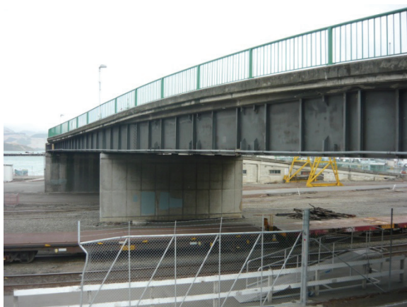
Figure 24 – Lyttleton Port Bridge (a) Plate Girder (b) Abutment Spalling (MacRae)
