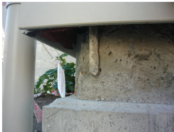
(a) Overall View from the South (b) Baseplate bolt at SE corner of the building Figure 19. Heathcote Valley Primary School Steel Moment Frame building (Photos: MacRae)
