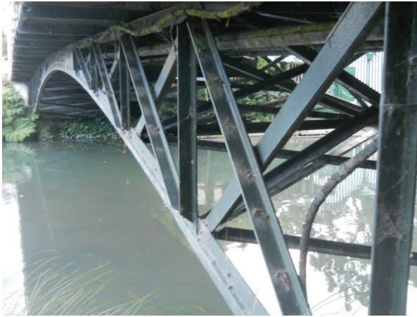
Figure 21 – Undamaged older steel pedestrian bridges on the Avon River near the CBD (Leon)
