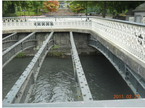
Figure 21 – Undamaged older steel pedestrian bridges on the Avon River near the CBD (Leon)
