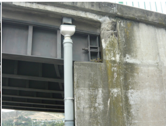
Figure 24 – Lyttleton Port Bridge (a) Plate Girder (b) Abutment Spalling (MacRae)
