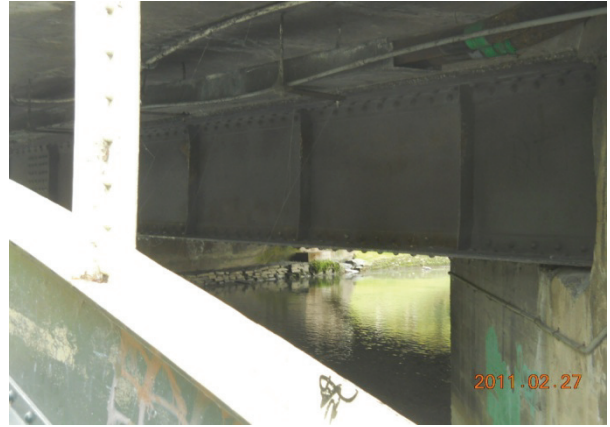
Figure 22 – Colombo Street bridge (a) Slumping of riverbank close to bridge; (b) Buckling of fascia arches; (c) Slumping of abutments at end of bridge; (d) Undamaged straight riveted girders. (Leon)
