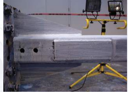
Brace Reinforcing – Structure Magazine
