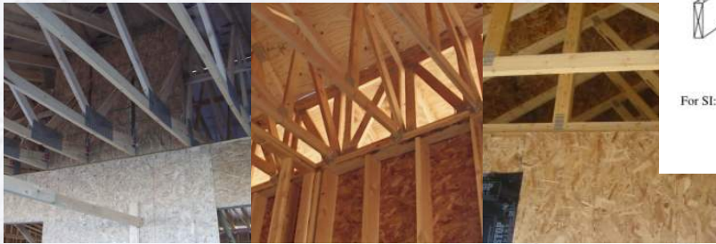
FIGURE R602.10.8.2(1) BRACED WALL PANEL CONNECTION TO PERPENDICULAR RAFTERS
